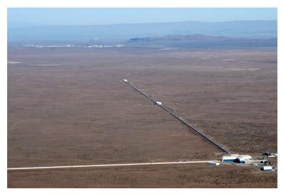
The LIGO detector in Hanford, Wash., uses lasers to measure the minuscule stretching of space caused by a gravitational wave. LIGO Laboratory
